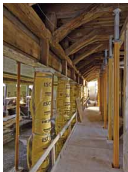
Hestestalden under renovering
